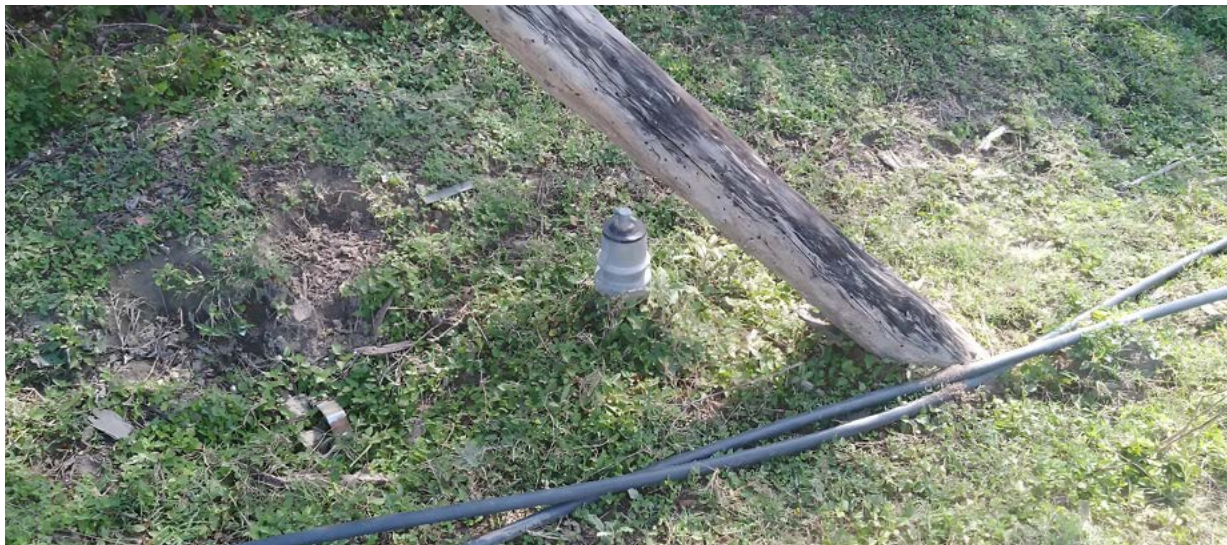
Photo 2. Gate valve in the pipeline
