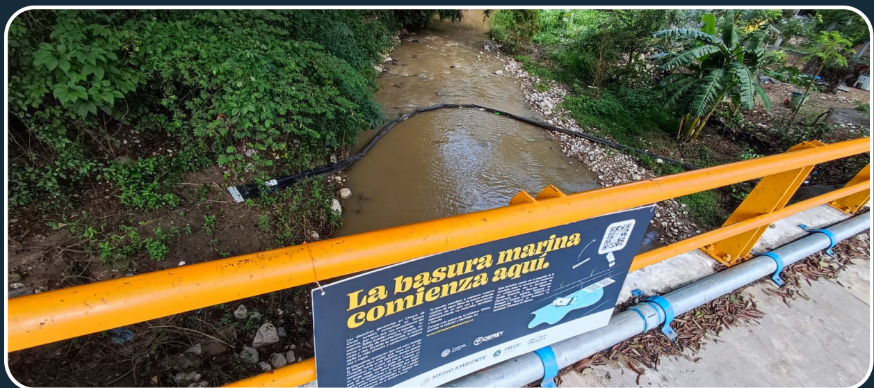
Trash capture devices, including the litter boom pictured above, were installed at three sites on the Rio Chiquito in Chiapa de Corzo at: Los Manguitos, Super Che, and Domingo Ruiz. Source: Osprey Initiative
