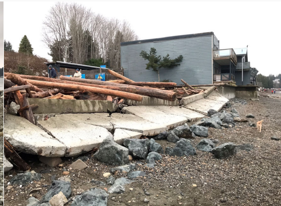
Figure 18. Photos of the shoreline following the 7 January 2022 storm, (left) along the restored creek estuary, and (right) along an adjacent section of shoreline, at which the seawall failed
