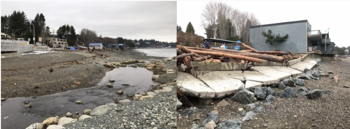
Figure 18. Photos of the shoreline following the 7 January 2022 storm, (left) along the restored creek estuary, and (right) along an adjacent section of shoreline, at which the seawall failed
