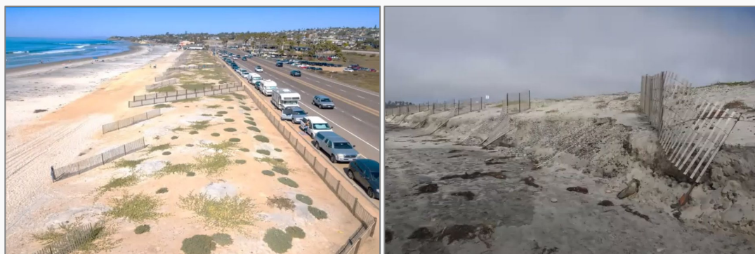
Figure 5. Dune construction after construction (left) and after two winter seasons of erosion (right)
