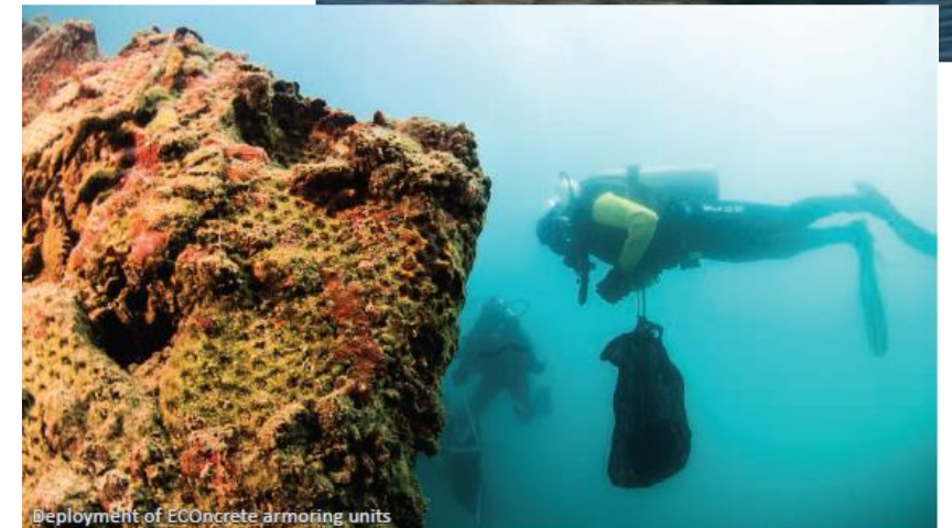
Deployment of EConcrete armor units
