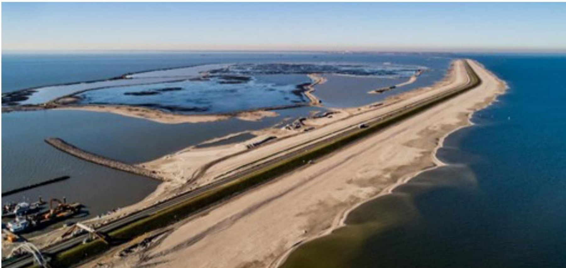
Sand Reinforcement of the Houtribdijk Dam
