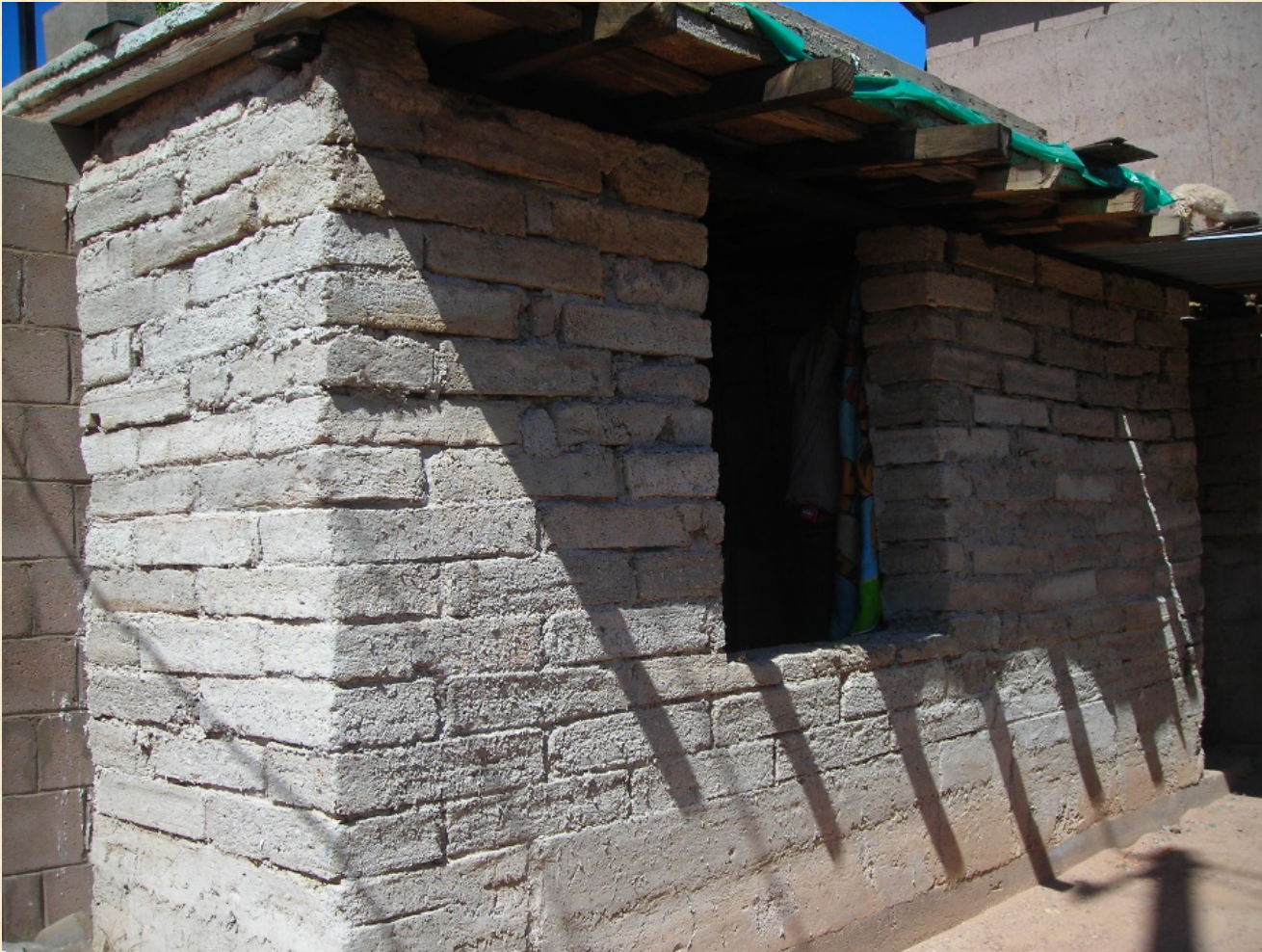
A two-room self-built fibrous concrete house under construction, Nogales, Sonora.
