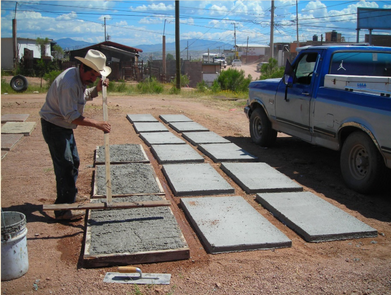
Fibrous concrete utilizing waste paper in the construction of housing for low-income families in Ambos Nogales.
