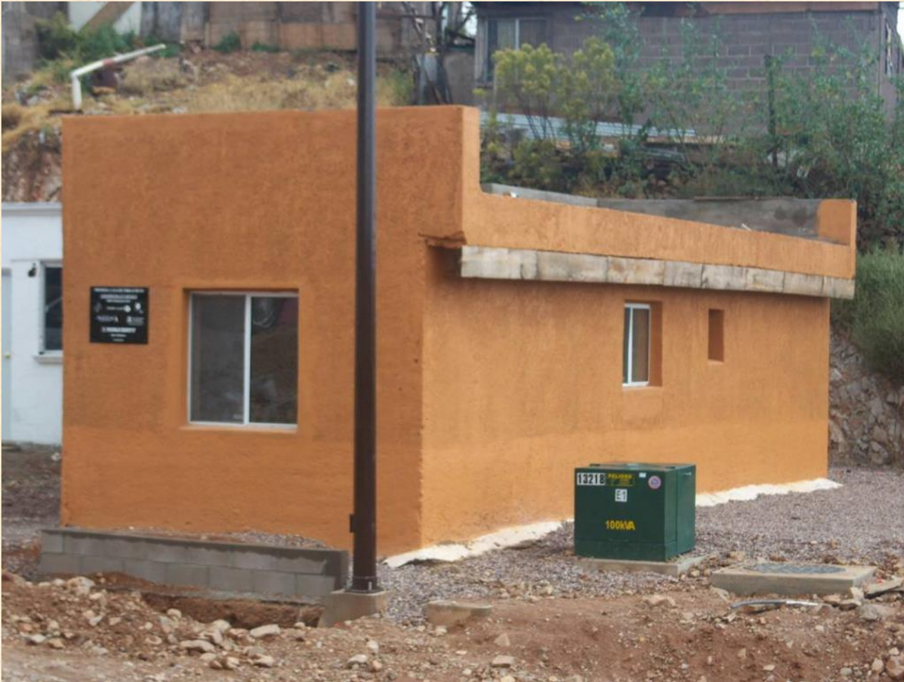
Completed Alcatel-Lucent fibrous concrete house, Nogales, Sonora.
