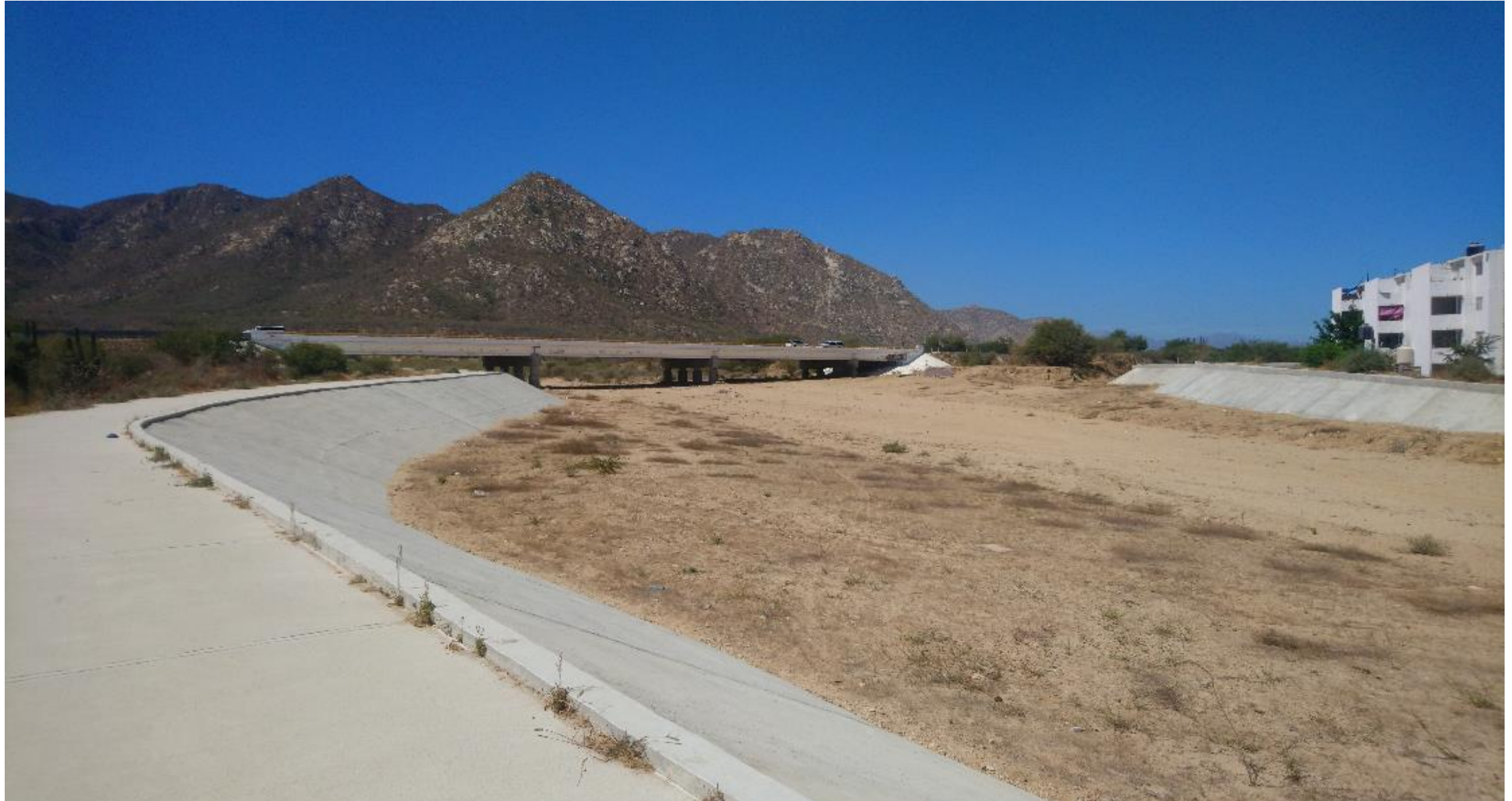
Implemented solution: containment for future flooding in Puerto Nuevo subdivision
