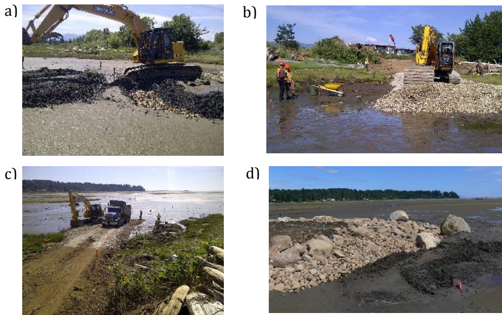
Figure 50. Construction of saltmarsh islands. a) Fill was added to allow movement of heavy equipment onto the mudflat; b) larger rock was incorporated at the front edge of each island; c) construction of the second island; d) detail of the front toe of the second island.
