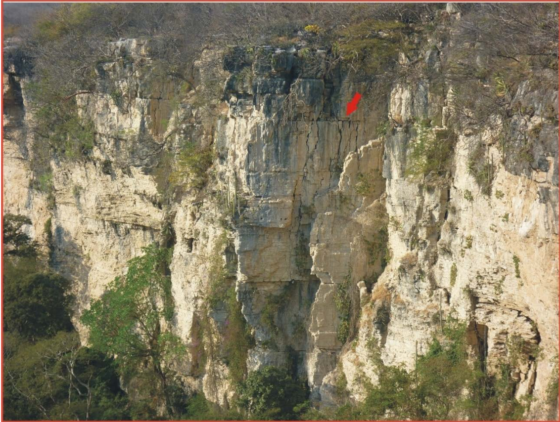
Figure 3: Cracks in the wall of Sumidero Canyon on the side where Cales y Morteros de Grijalva, S.A. de C.V. is operating. Source: Our photo.
