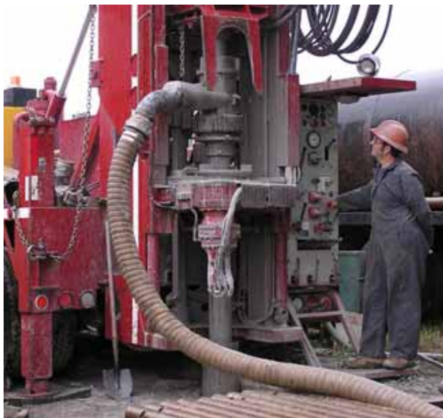
Figure 4.2 Installing a Groundwater-Monitoring well.
