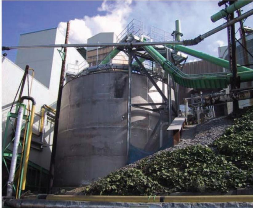
Figure 13. Irving Pulp and Paper Mill – MBBR (photo courtesy of Irving)
