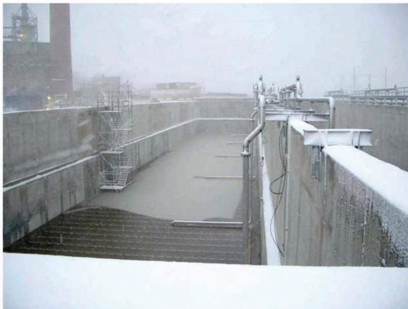
Figure 5. Aeration Basins for AST System at ACI Mill
