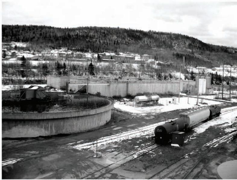
Figure 16. Clarifiers and Oxygen Reactor, AV Cell Mill
