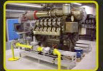
ELECTRICITY GEN. FROM METHANE
