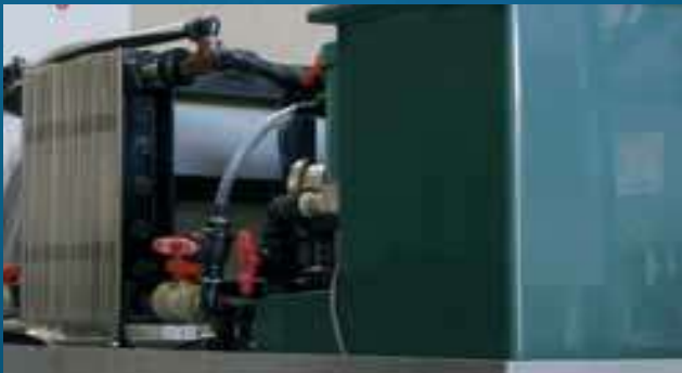
Figure 2: A 1-10 kWh VRB installed by UNSW in a Solar Demonstration House in Thailand in the mid-1990s (top) and 5 kWh VRB lab test battery (bottom).
