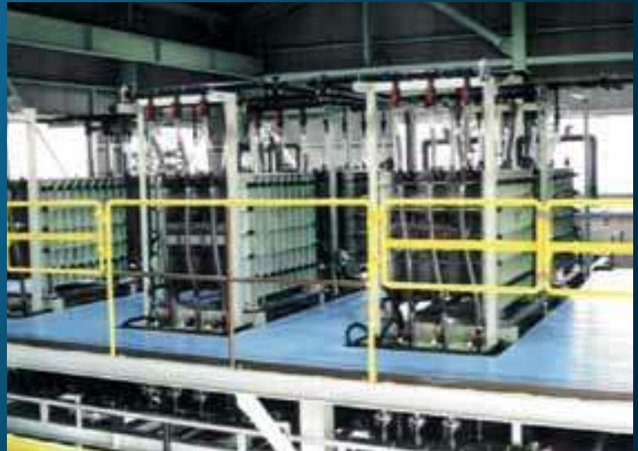
Figure 4: 200 kW/800 kWh VRB installation at the Kashima-Kita Electric Power station in Japan (installed in the mid-1990s).
