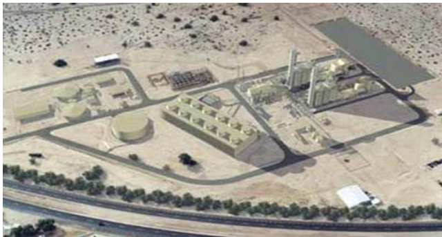
Termoelectrica de Mexicali (625 MW natural gas combined cycle power plant in Mexicali)
