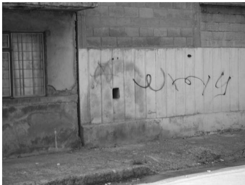
Photo No. 2: Zone for delivering of solvents (xylene and styrene), next to Submitter's residence on 11 Cerrada de Vaqueros . There is a hole in the wall for inserting a hose used to deliver the product.
