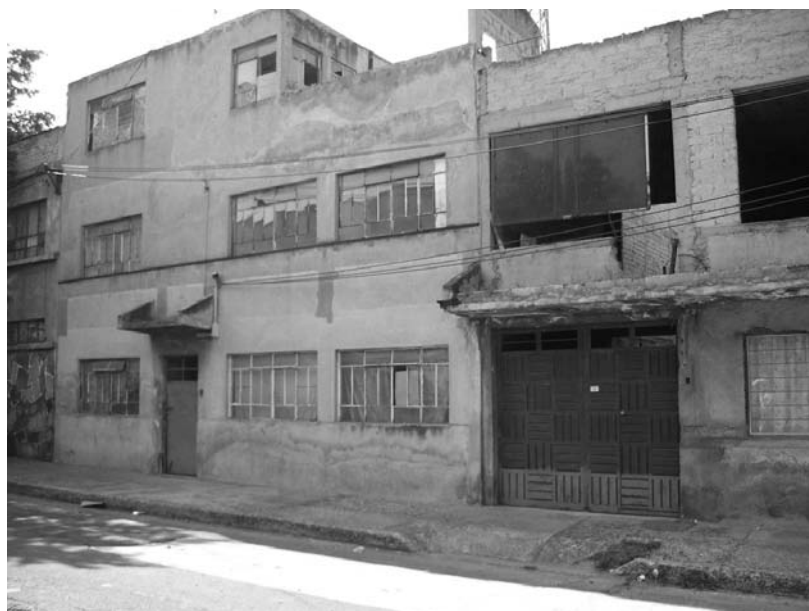
Photo No. 1: View to the west of Submitter's residence, located at 11 Cerrada de Vaqueros street.
