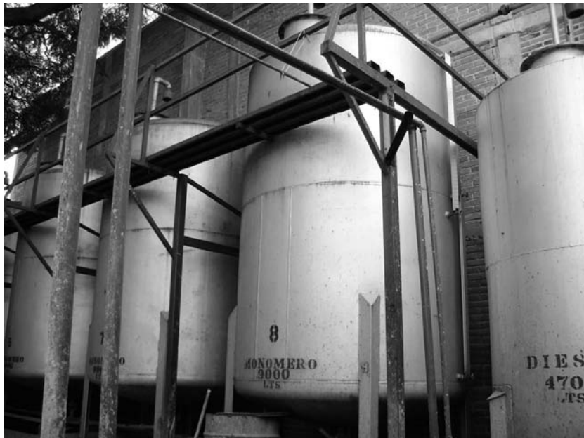
Photo No. 4: Area with storage tanks for chemical products. There are no signs indicating the presence of risk. At the back of the area is the wall bordering the Submitter's residence.
