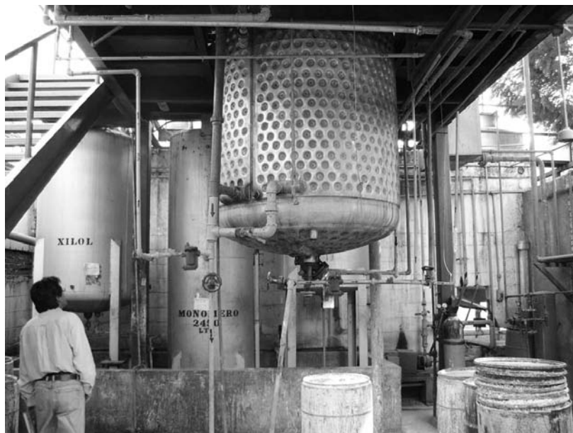
Photo No. 5: Reactor used to produce latex. The drums were used for transporting the product to the saturation area. Day tanks for xylene and styrene monomer can be seen at the back.
