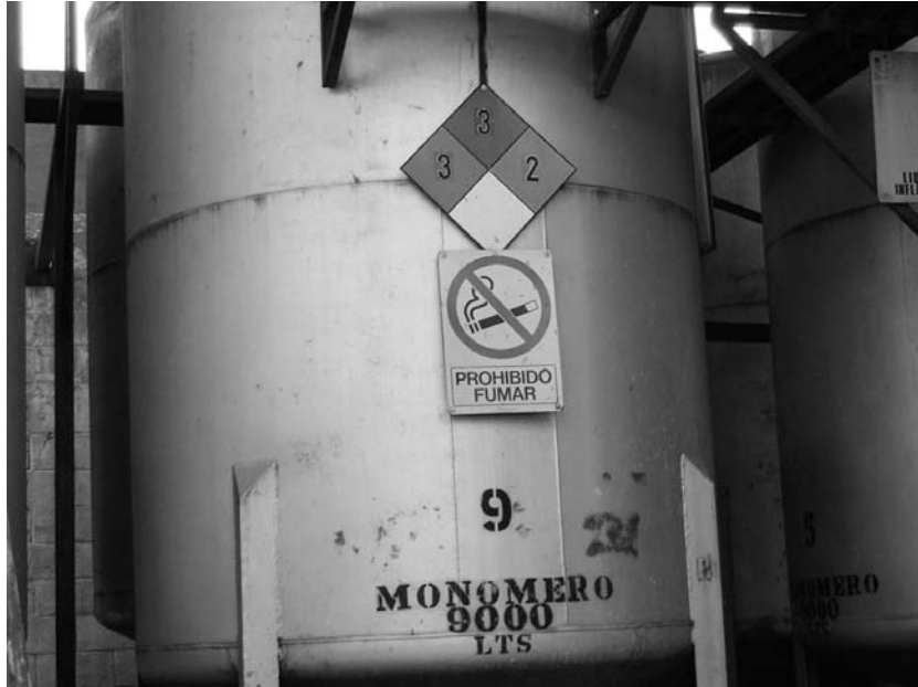
Photo No. 3: Styrene monomer storage tank with capacity of 9,000 liters. Only some of the tanks were observed to have the corresponding indications.
