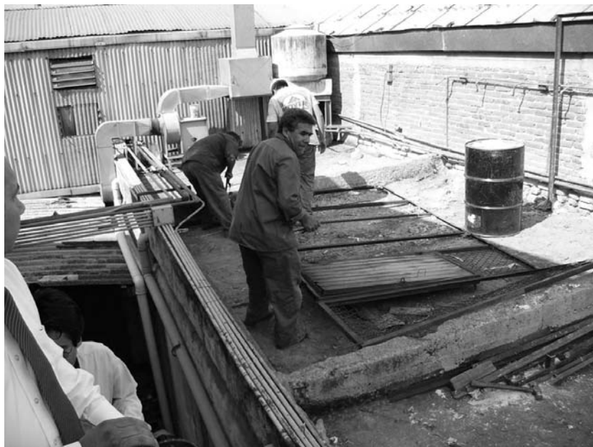
Photo No. 10: Dismantling of the ALCA's facility.
