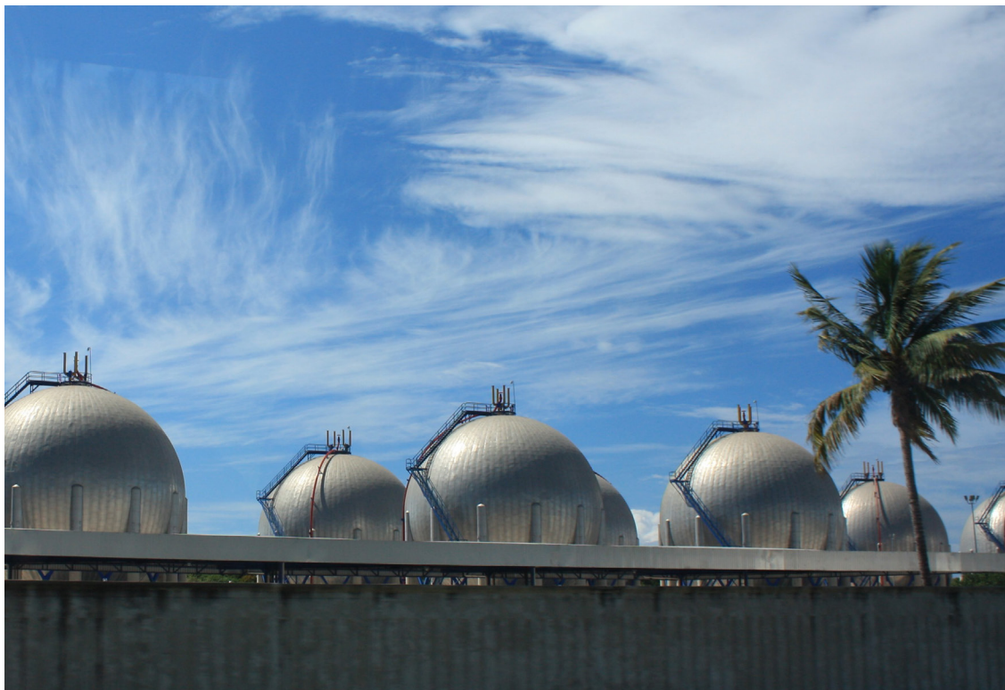
Photo 2: Terminal Gas LP Manzanillo
