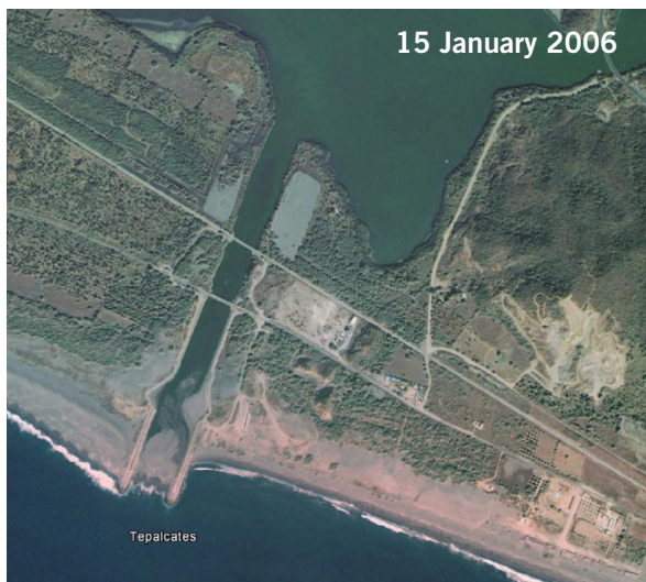
This photo clearly shows net transport of sand toward the east, with accretion of sand behind the west breakwater.
