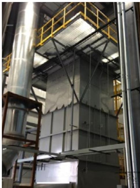
Fuente: Envitech Inc. (s/f), “Wet electrostatic precipitator (WESP)”, en: <[www.envitechinc.com/wet-electrostatic-precipitator/](http://www.envitechinc.com/wet-electrostatic-precipitator/)>.
