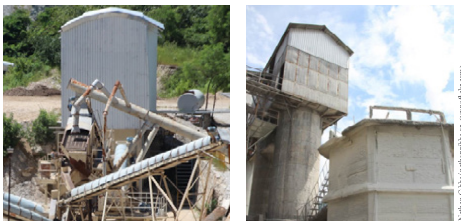
Photo 5. Enclosure of production facilities 286
