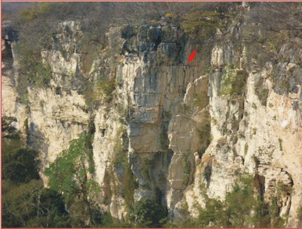
Figure 3: Cracks in the wall of Sumidero Canyon on the side where Cales y Morteros de Grijalva, S.A. de C.V. is operating. Source: Our photo.
