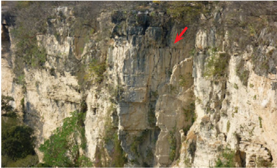
Photo 6. Cracks in the east wall of Sumidero Canyon 325
