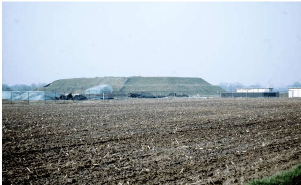
Photo 2. This photo from the mid-1990s is of a temporary storage site in the Netherlands for 200,000 tons of soil contaminated with waste HCH isomers.
