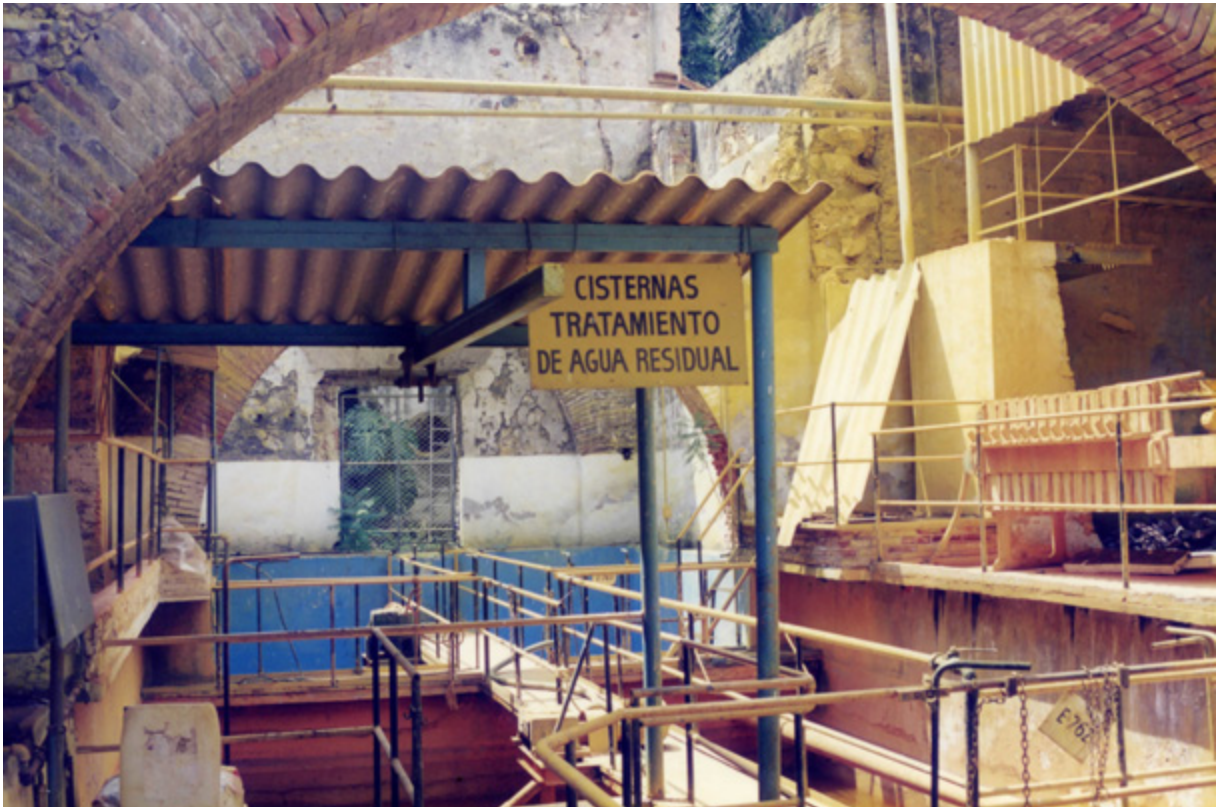
Photo 3. Wastewater treatment plant of the Facility 371
