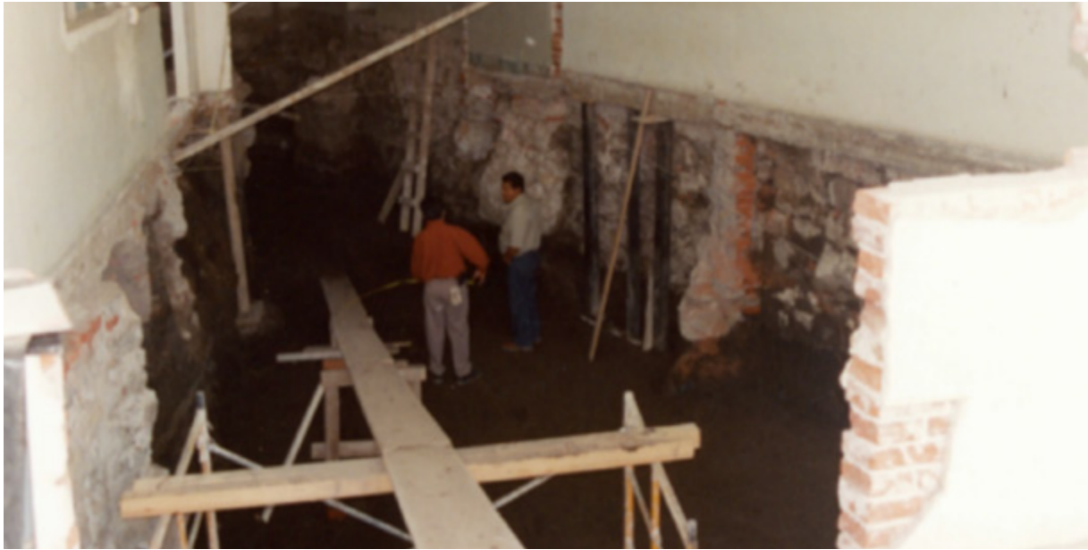
Photo 7. Excavation in the offices area 718
