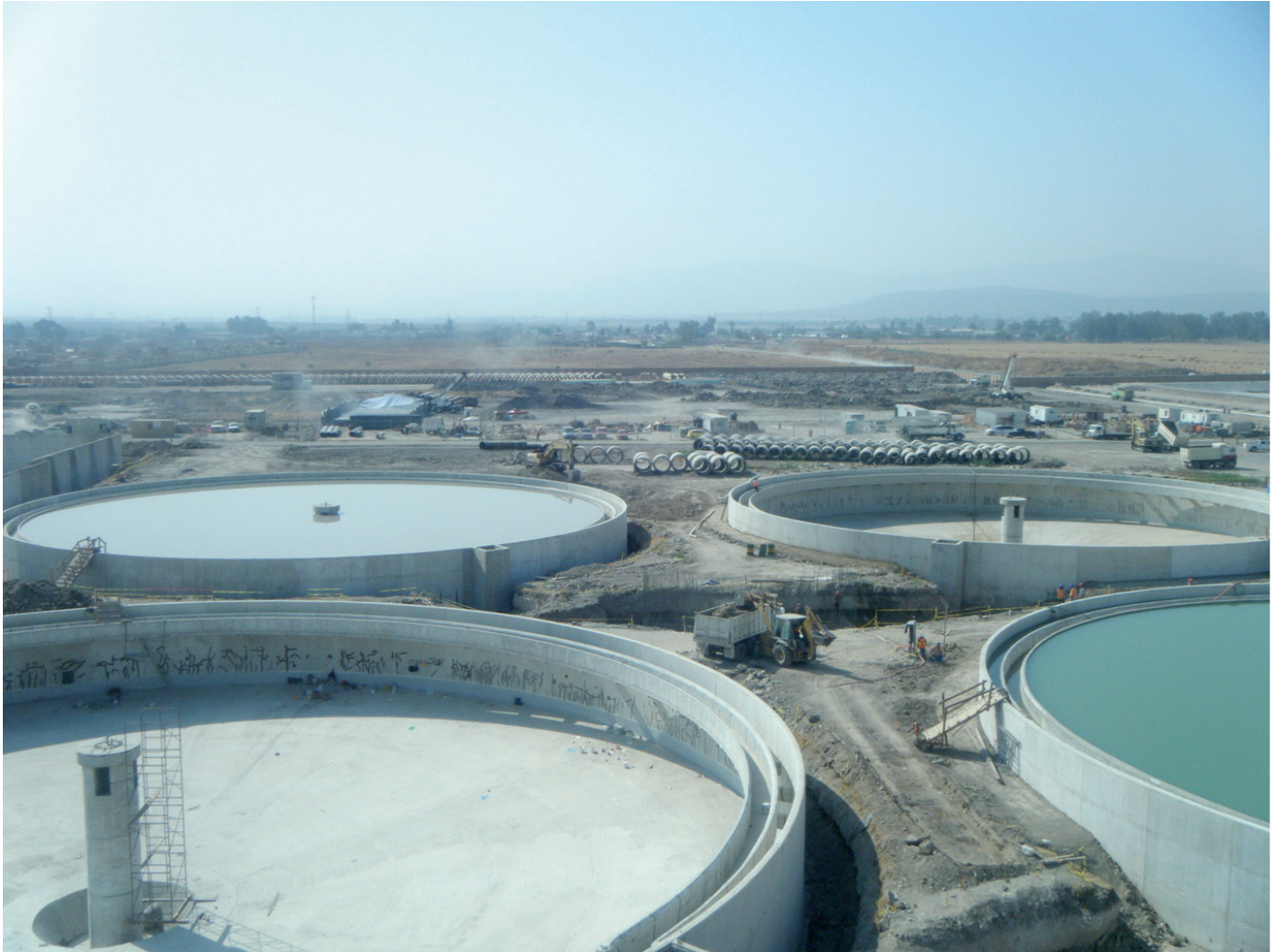
Photo 3: View of the El Ahogado wastewater treatment plant under construction 559
